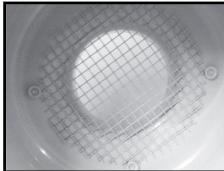
Step 17. Check inlet grille is clear.
